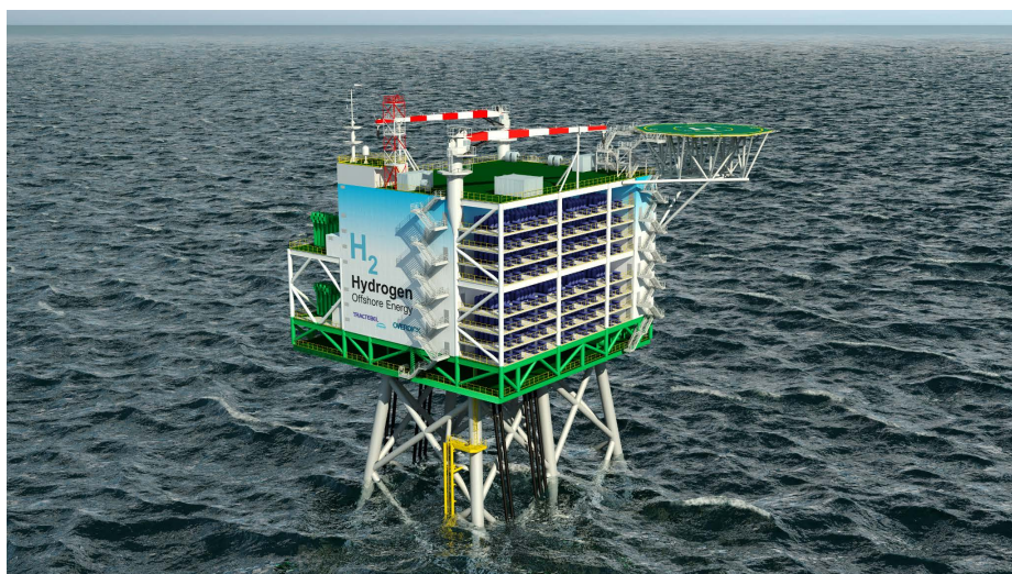
Image 2: Offshore Electrolyser (from Tractebel)
