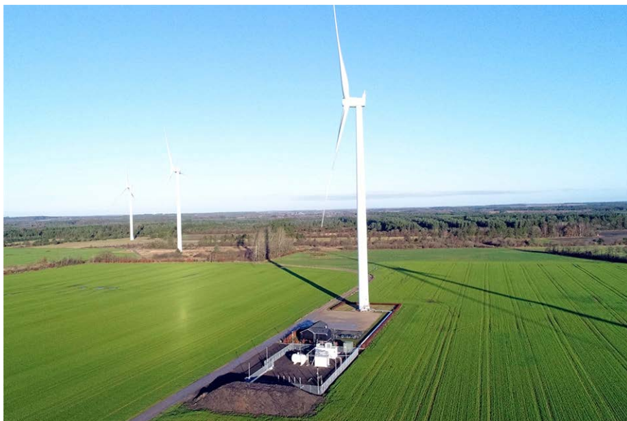
Image 1: Behind-the-Meter Electrolyser (from Siemens Gamesa)
