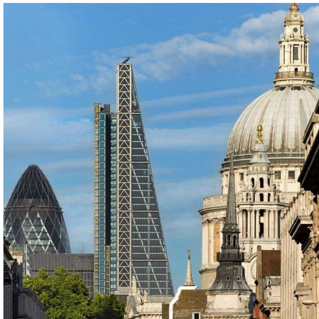
Fig. 1.11 The Leadenhall Building's distinctive slant was an architectural response to the LVMF's demand that it avoid intruding on one of the viewing corridors centred on St. Paul's Cathedral
