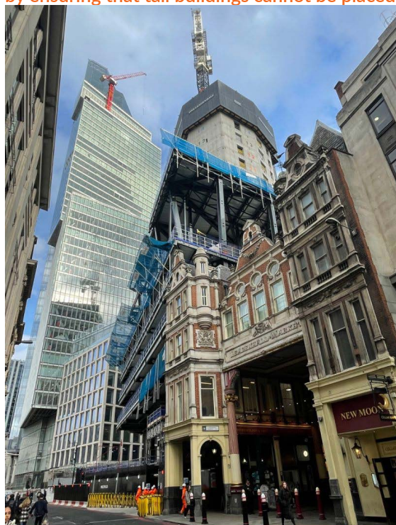
Fig. 2.6 The Leadenhall Rule will maintain the historic integrity of listed buildings by ensuring that tall buildings cannot be placed directly beside them
