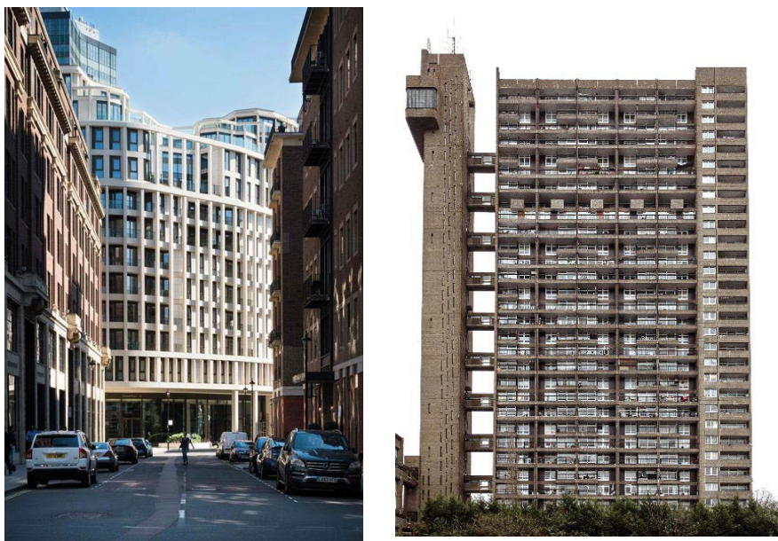
Fig. 2.18 & 2.19 Despite being almost three times shorter than Erno Goldfinger's infamous Trellick Tower in London's North Kensington, modern Westminster mansion blocks Abel & Cleland Houses are 2.1 times as dense
