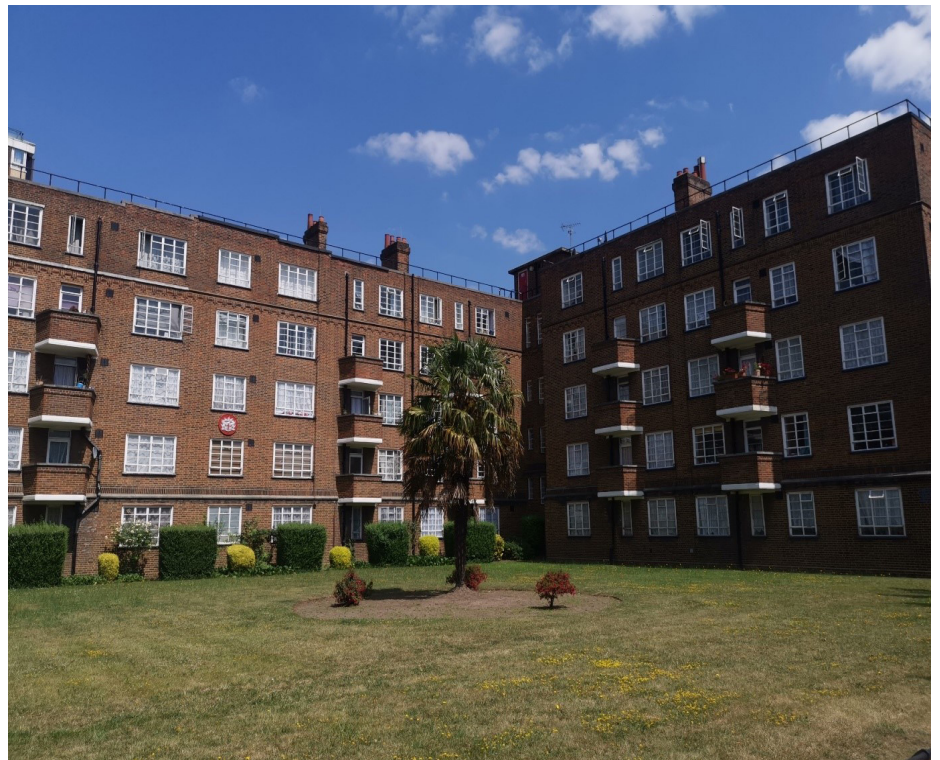
Early 20th century social housing models sought to seamlessly integrate balconies into their masonry elevations rather than express them as architecturally distinct additions, thereby helping give the developments an reassuring sense of mass and solidity.
