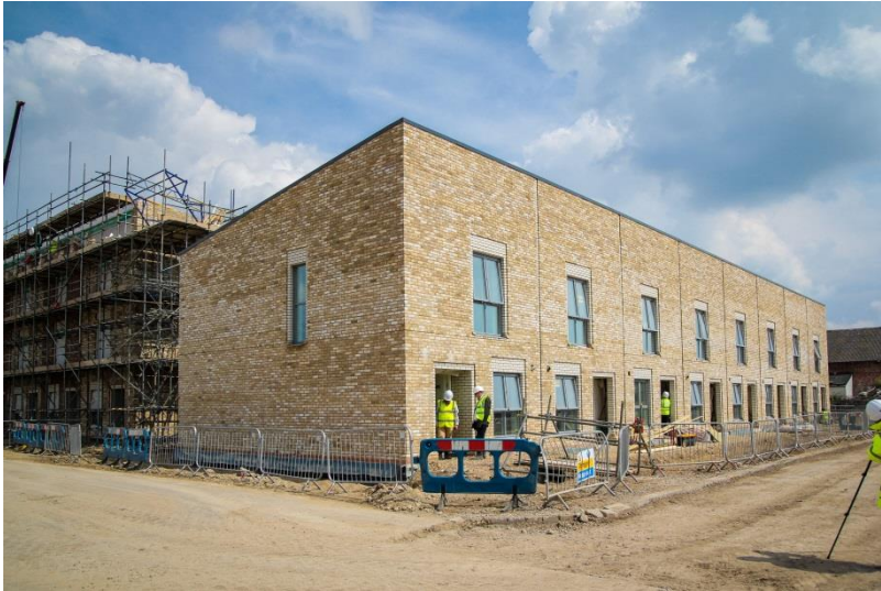
Apartments constructed with manufactured concrete panels, Barking
