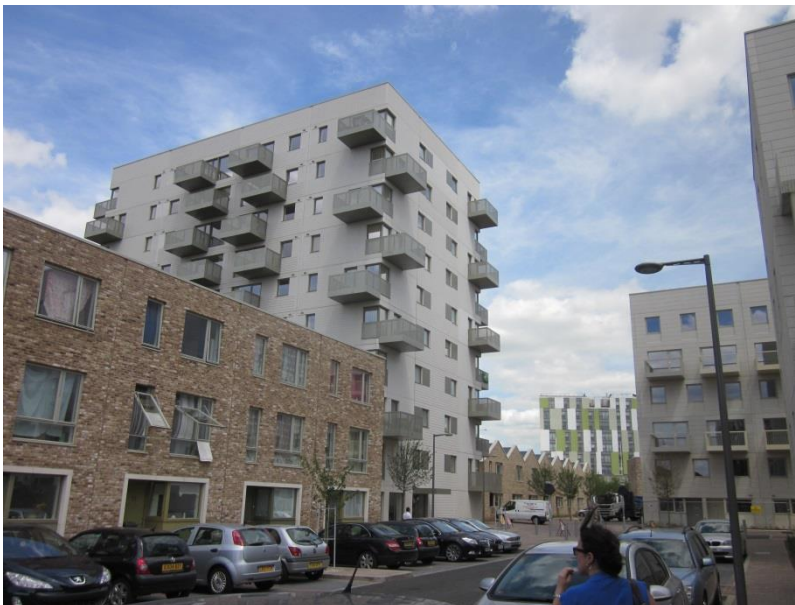
Apartments constructed with manufactured concrete panels, Barking
