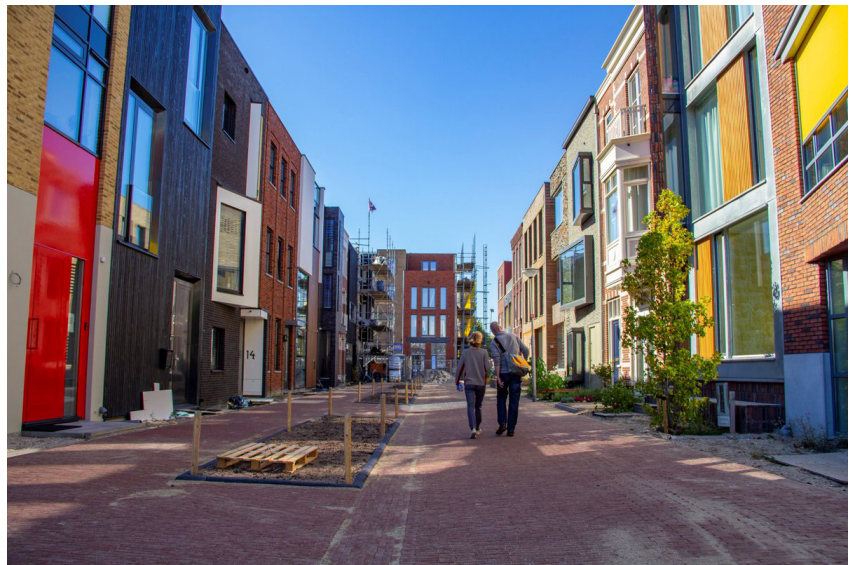
A modern terraced street in Delft, still under construction. Credit: Graham Taylor, taylorcreations.co.uk .
