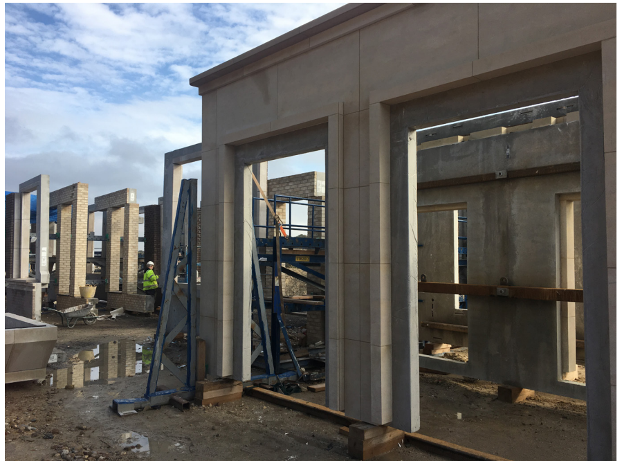
Brick and stone wall panels constructed off-site. Credit: author.
