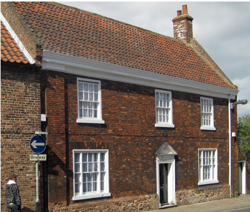
Design features like exposed brickwork is valued by people. Source: David Wright, Flickr (Creative Commons).
