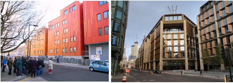
Left: Fibre cement cladding on a residential block in London. Credit: Steve Cadman, Flickr (Creative Commons). Right: The Bloomberg European HQ (Foster + Partners, 2018) uses cladding systems but with natural materials such as stone and wood. Credit: ACME, Flickr (Creative Commons).
